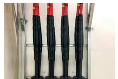
24CSJA-S cold-shrinkable straight joint
