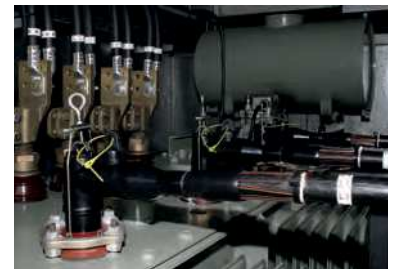
Transformer connection with 158LR
