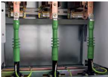
AIS20 with mechanical cable lug
