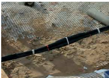
TS-24CSJ hybrid transition joint
