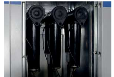
SF-6 system connection with 480TB+800SA
